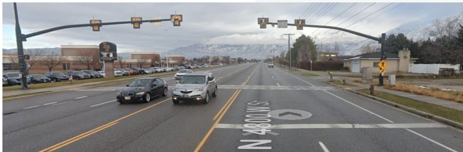
Pedestrian Hybrid Beacon Accessing Lone Peak High School on North County Blvd, Highland
