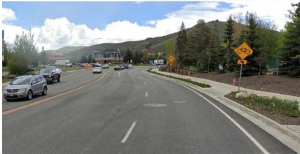
Providing early access to a paved path or sidewalk can remove some of the complexity of the interface between a right turn lane and the bike lane (Example: SR-224 in Park City)
