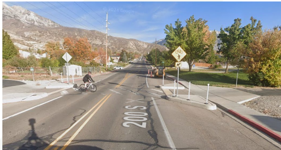
Murdock Canal Trail Crossing 200 S in Lindon – Bulb-outs assert the right-of-way for trail users and decrease crossing distance.
